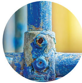
Pipes and hardware
