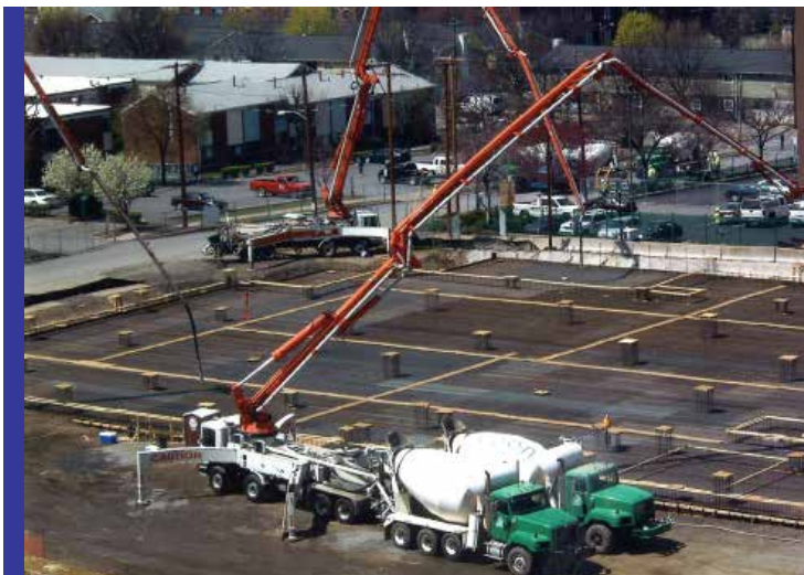
The west side of the building is built on pylons.
