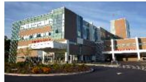
Geisinger Wyoming Valley Critical Care Tower
