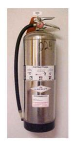
Class A fire extinguishers can be used on wood, paper, textiles, and rubber ONLY
