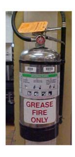
Class K fire extinguishers can be used on high temperature fires involving burning cooking fats and oils
