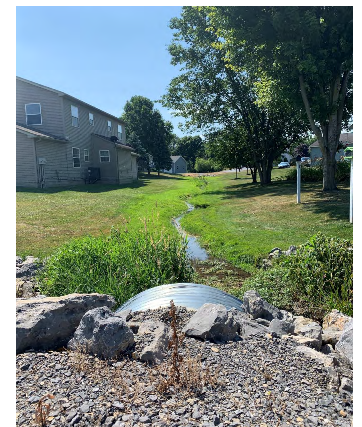
Figure 4. Image of a culvert in Buffalo Creek at Gessner Lane
